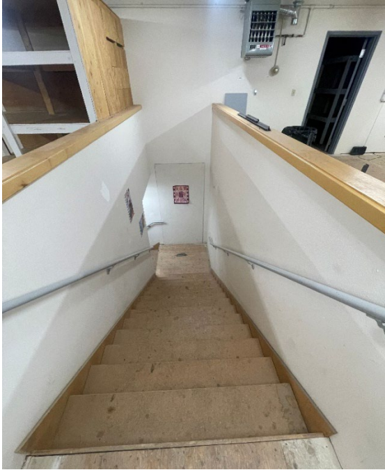
Figure 1.2 - Former Warehouse – Stairway – View up
