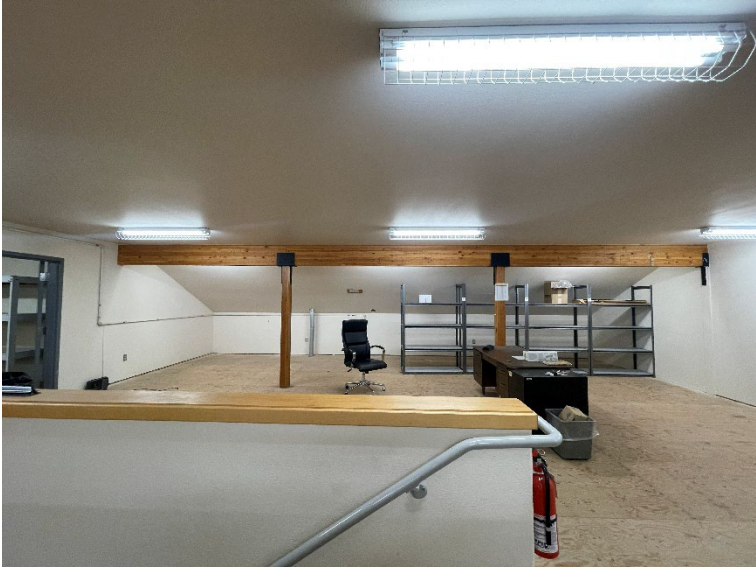
Figure 6 - Former Warehouse – Southside.
